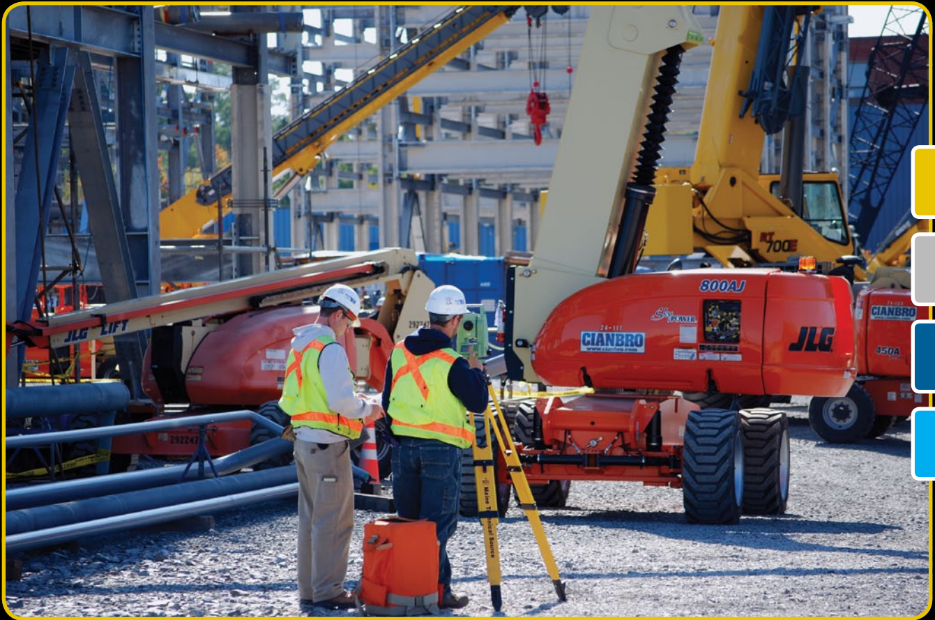
At every position, field crews scan about one-quarter of a module depending on the module's size in about 15-30 minutes, gathering some 1.5 million points per set-up.
